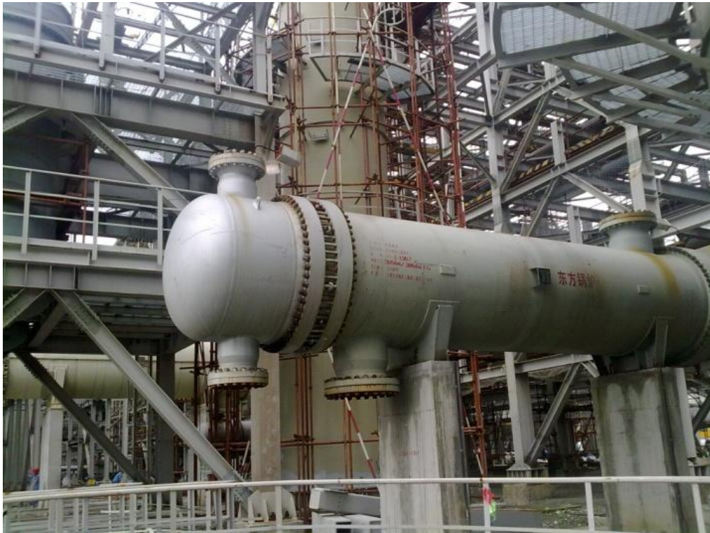
Floating-head heat exchanger for Pengzhou Petrochemicals 800000 tons/year ethylene project under installation
